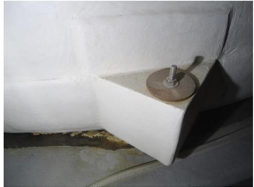
Photo Set 2: Tank hold down lugs: appear to be structurally sound
