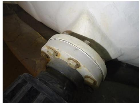
Photo Set 3: Tank manway & fitting flanges (outside) – no issues
