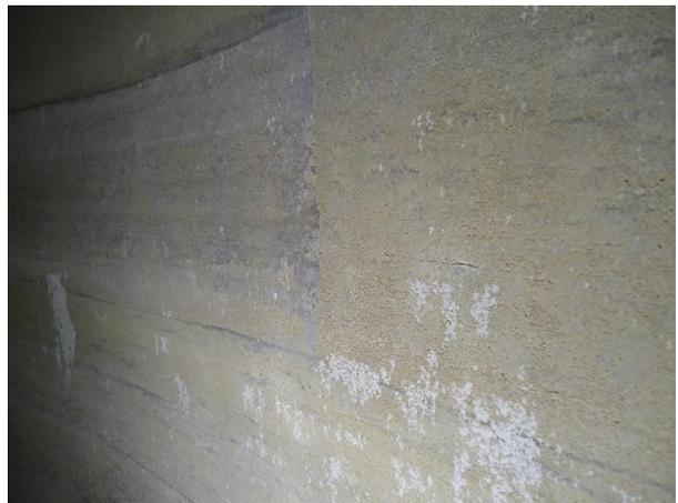
Photo Set 10: Close up view of the dryness and roughness of the tank wall
