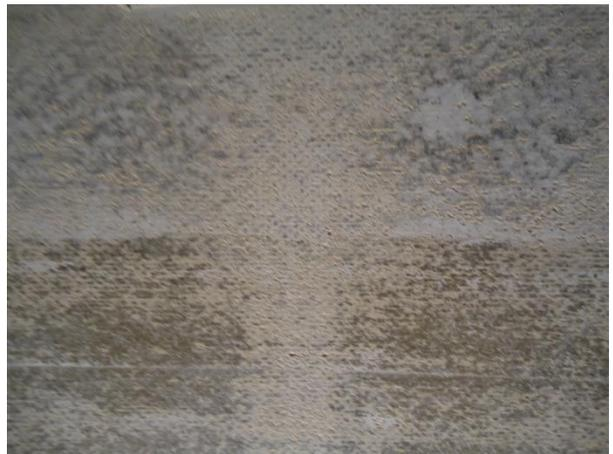
Photo Set 11: Close up view of the dryness and roughness of the tank wall
