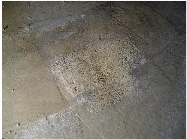
Photo Set 9: Close up view of the dryness and roughness of the tank floor
